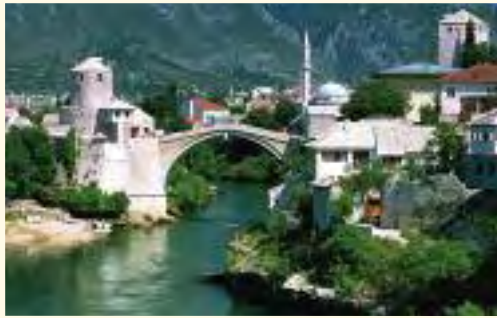
Mostar's restored 16 th -century Ottoman Stari Most Bridge connects Bosnia with Herzegovina.
