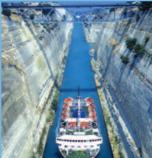
Admire the spectacular 300-foot sheer cliff walls of the Corinth Canal as you navigate this engineering marvel.
