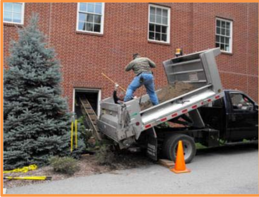
The first load of sediment in September.
