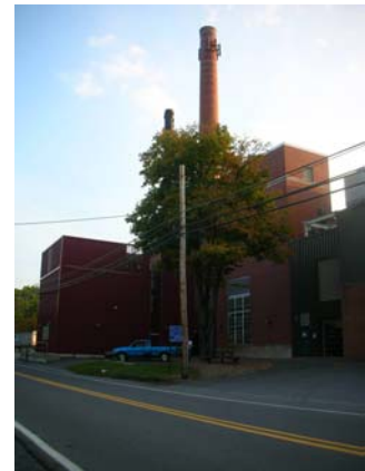
Figure 1. The co-generation plant on Bucknell's campus. Produces the majority of electricity used at Bucknell. C. Kassab
